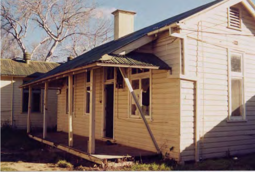
Plate 18: Block J - demolished (JAA 1996)
