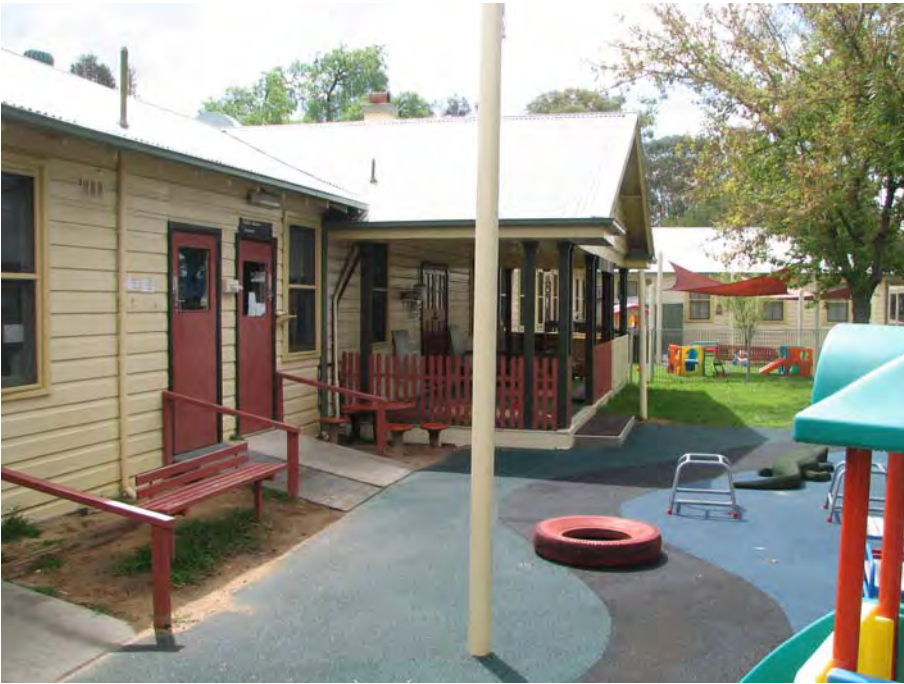
Plate 8: F Block; east side. This aesthetically important elevation is obscured from view by E Block (JAA 2007)
