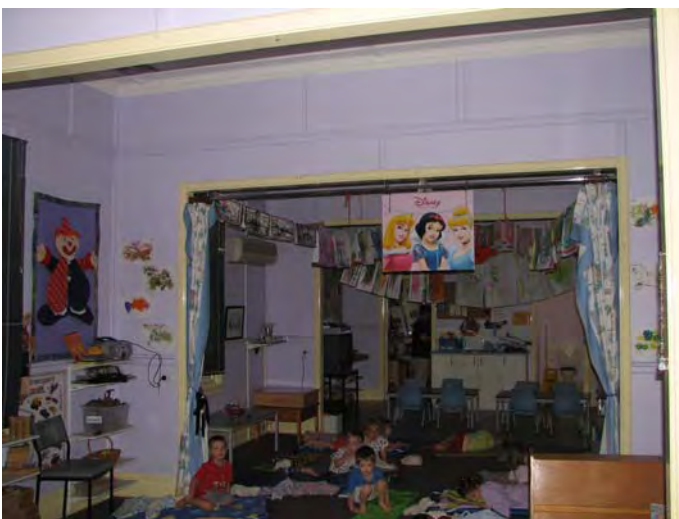
Plate 38: Block D; interior view showing nib walls and bulkheads to identify former individual bedrooms (JAA 2007)
