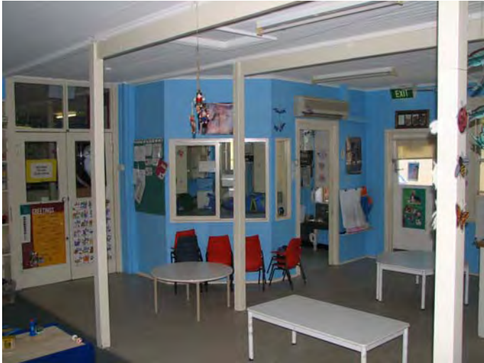
Plate 39: Block F. large interior spaces have been formed with the removal of inner walls. The posts and some bulkheads remain to identify the earlier configuration of rooms (JAA 2007)
