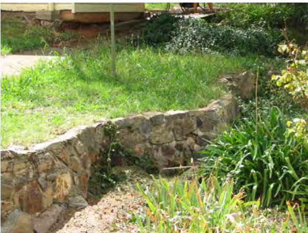
Plate 32: Retaining wall used as building platform for Block L (demolished) (JAA 2007)
