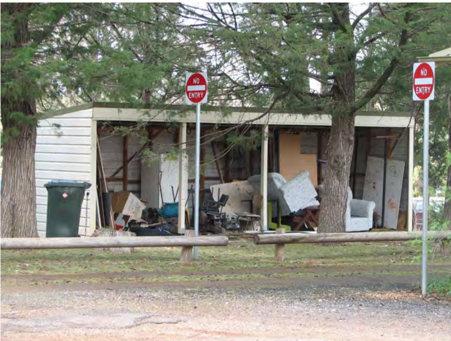
Plate 3: Bicycle shed (built to support residents/users of A Block (JAA 2007)
