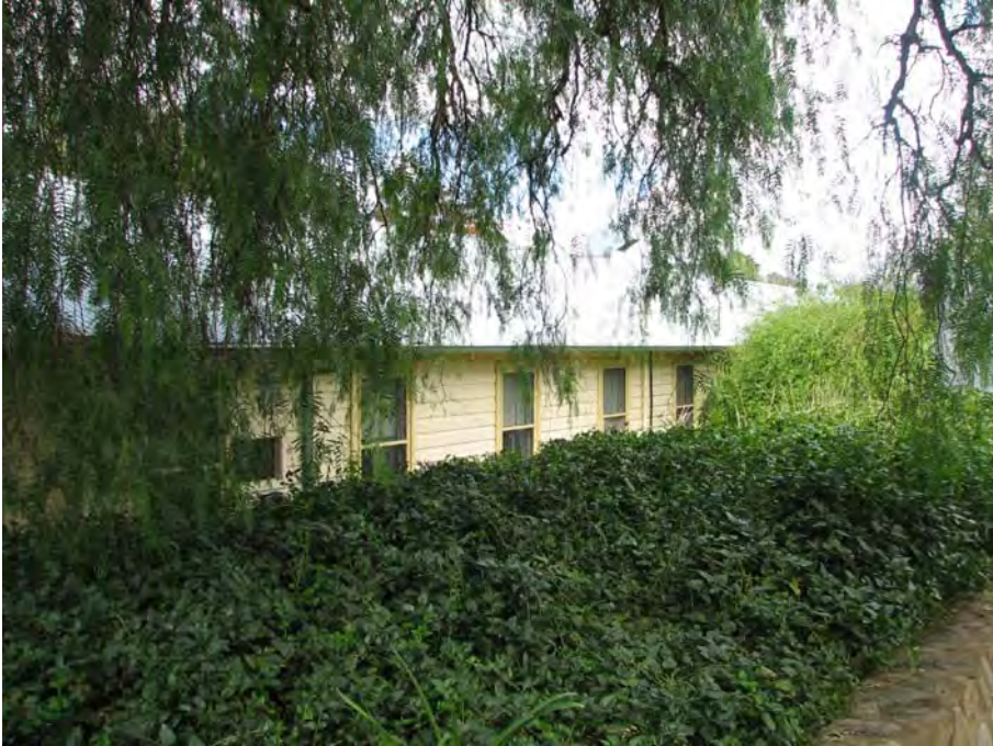
Plate 10: F Block; west side. The remnant stone wall under the overgrowth has heritage significance (JAA 2007)
