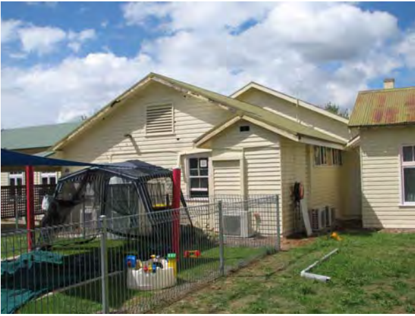
Plate 33: Block G; west view, with play equipment in foreground (JAA 2007)
