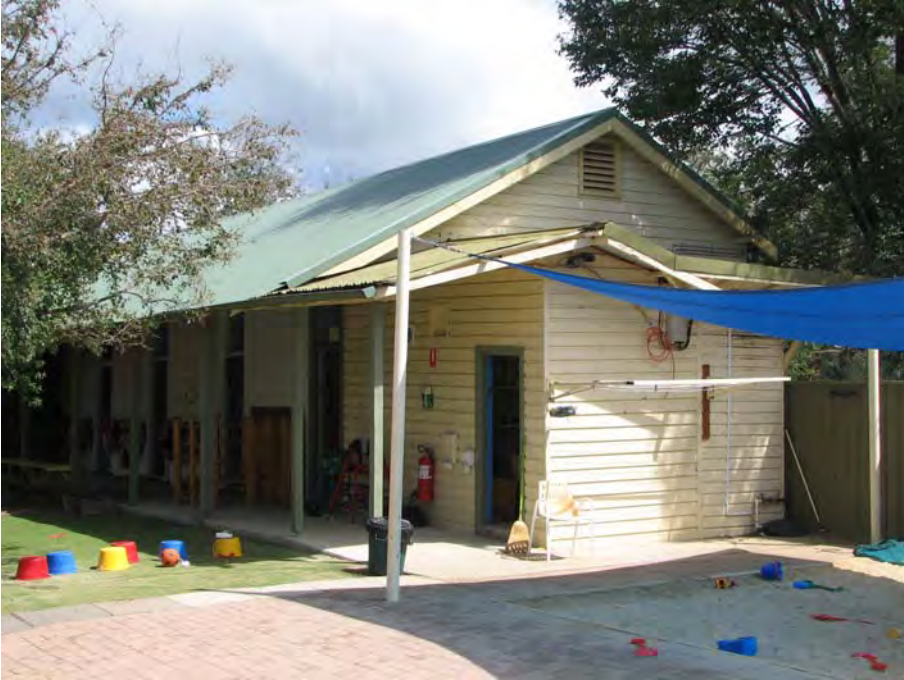
Plate 4: D Block; north side. Note replacement roofing (JAA 2007)
