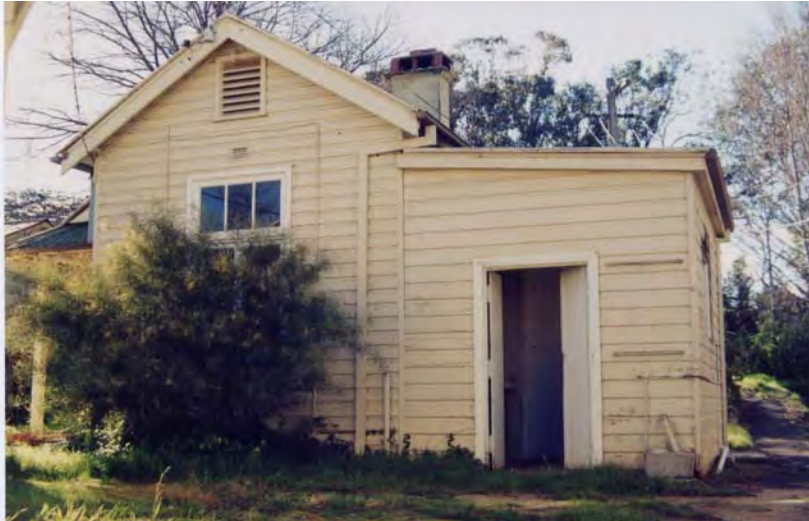
Plate 19: Block K - demolished (JAA 1996)
