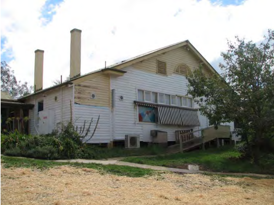
Plate 11: G Block; east side. This elevation was built in the late 1920s (see Plate 1 for original appearance) (JAA 2007)
