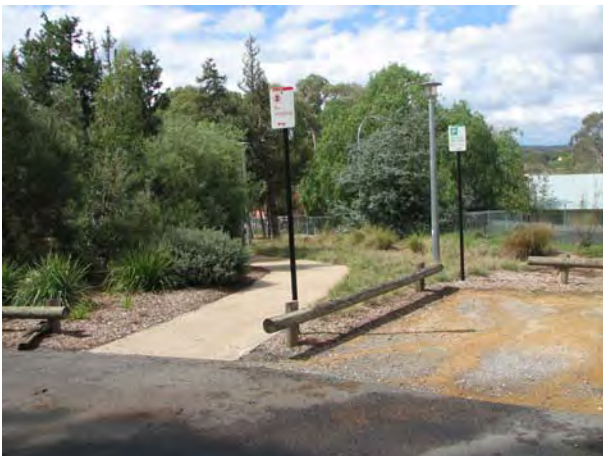
Plate 29: Path leading from north carpark down to Blocks E & F (the ANT Pres-School and Child Care Centre). Ramped access is a compliance requirement (JAA 2007)
