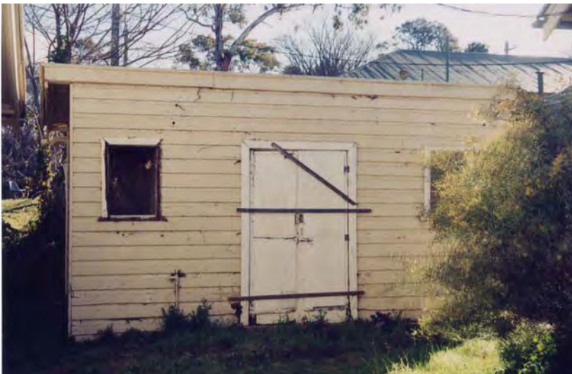
Plate 20: Block M - demolished (JAA 1996)
