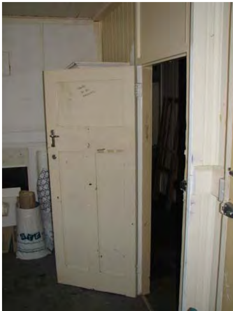
Plate 56: Block A. Typical high-waisted bedroom door with three panels. Note the door jamb is expressed and has the dual function of wall frame and door jamb. These functions would normally be provided with two separate timbers (JAA 2007)
