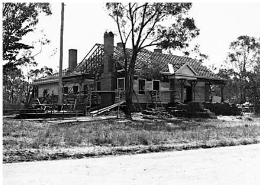
3 Liversidge Street under construction, 1927 (NAA A3560, 2793)
