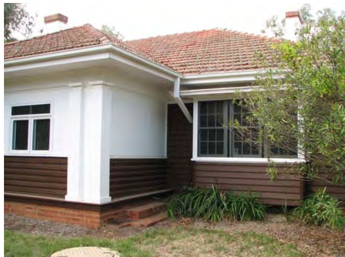
Figure 4.40: The north verandah (above) and western verandah with bay window.
