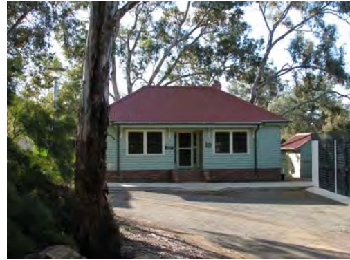
Chauffeur's Cottage in new location, view north (front)
