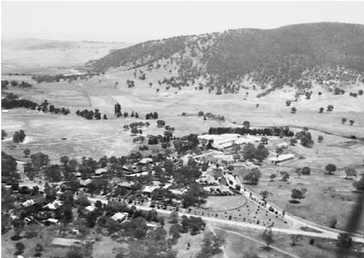
Figure 4.26: View southwest of the Balmain Crescent subdivision, 1928. The Acton Hospital can be seen in the background (NAA A3560, 7719).
