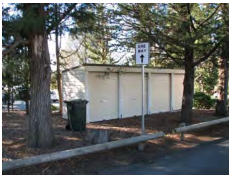
Bicycle/storage shed to the north of the complex (recent structure)
