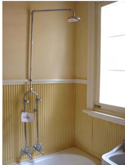
Figure 4.29: Intact features of the kitchen and bathroom
