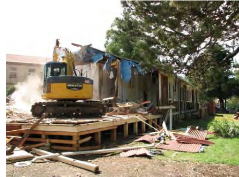
Demolition of B Block, Dec 2010
