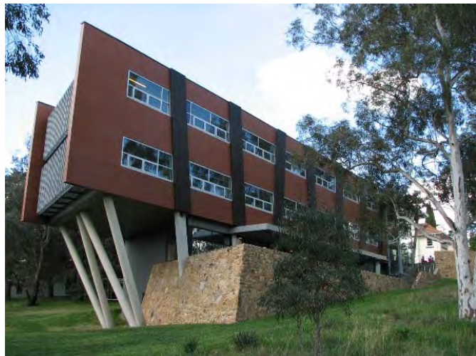
Figure 4.19: The southern end of the Crawford Building, 2010, located to the southwest of Old Canberra House
