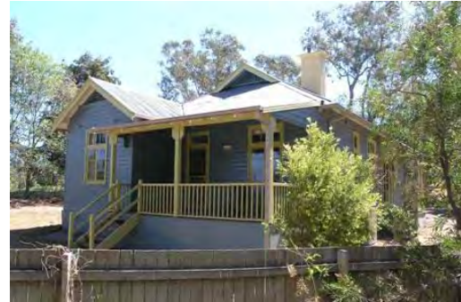
View west of 8 Liversidge Street, 2009
