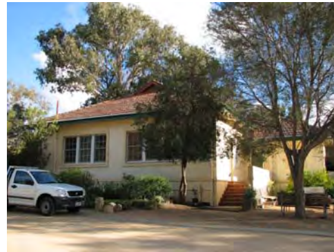
Gardener's Depot (office block), 2009
