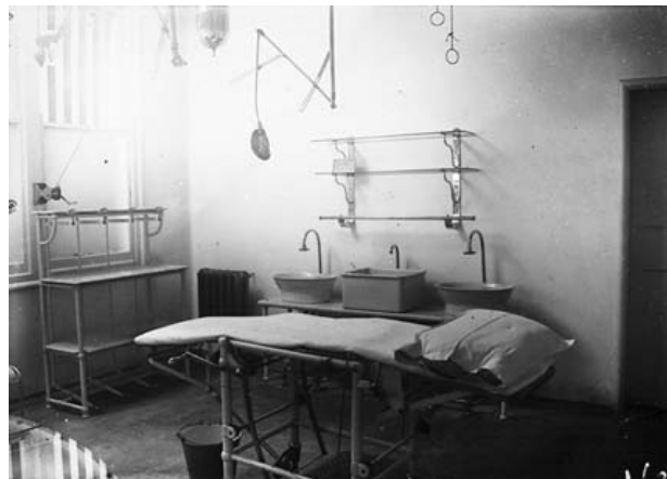
Figure 4.56: Operating Theatre, April 1926 (NAA A3560, 1630).
