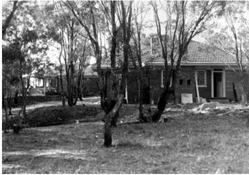
Construction of 14 Balmain Lane, c1926 (NAA A3560, 1842)
