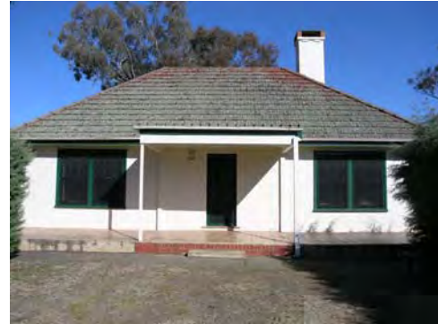
Gardener's cottage, view south (rear)
