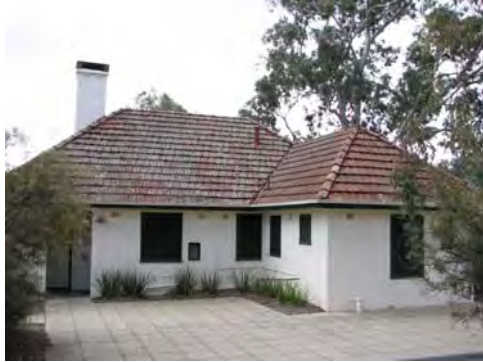
Gardener's cottage, view north (front)
