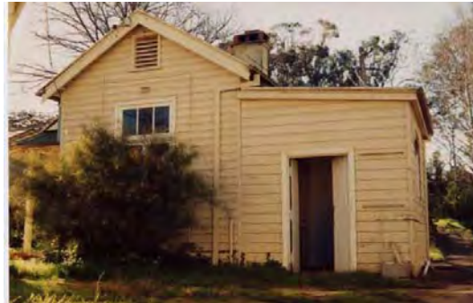
K Block prior to demolition (Armes 1996)
