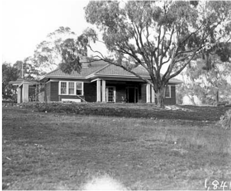
Construction of 16 Balmain Lane (NAA A3560, 1841)
