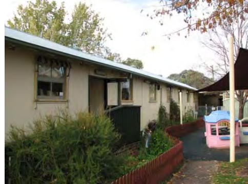
East side of E Block
