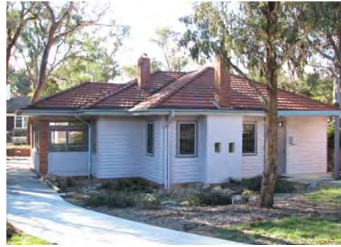
View north of 14 Balmain Crescent, 2009
