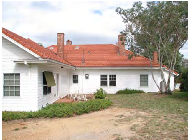
Figure 4.49: Rear courtyard formed by the northern extension.
