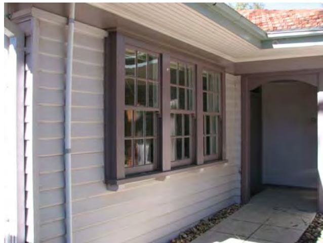
Figure 4.36: Two important features of the western façade are the enclosed verandah (above) and late Federation period 'triple' window (below).
