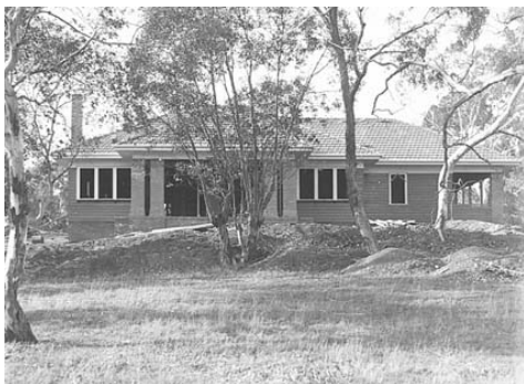
20 Balmain Lane under construction, 1926 (NAA A3560, 1644)
