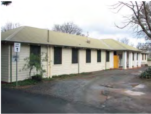
A Block (view SE), 2009
