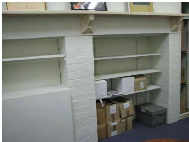
Figure 4.50: A common element to the Acton Cottages: the fireplace (kitchen range) converted into shelving.
