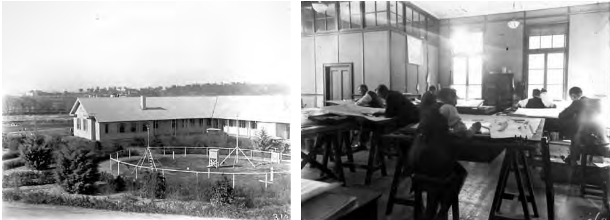
Figure 3.3: The Acton Administration Offices, seen here in the early 1920s, were the first supplied to Commonwealth employees in the Capital (NAA A3560, 314; A3560, 268).
